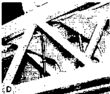
Pins and retainer pins installed to secure tip of Side Fly to rear support bracket
