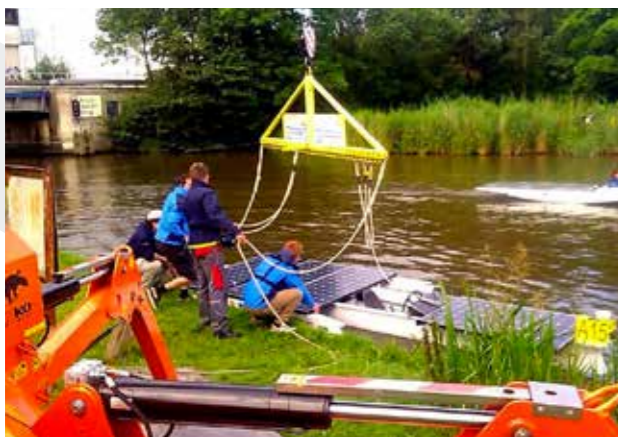
SPX527, installation of photovoltaic panels on a boat, ITALY
