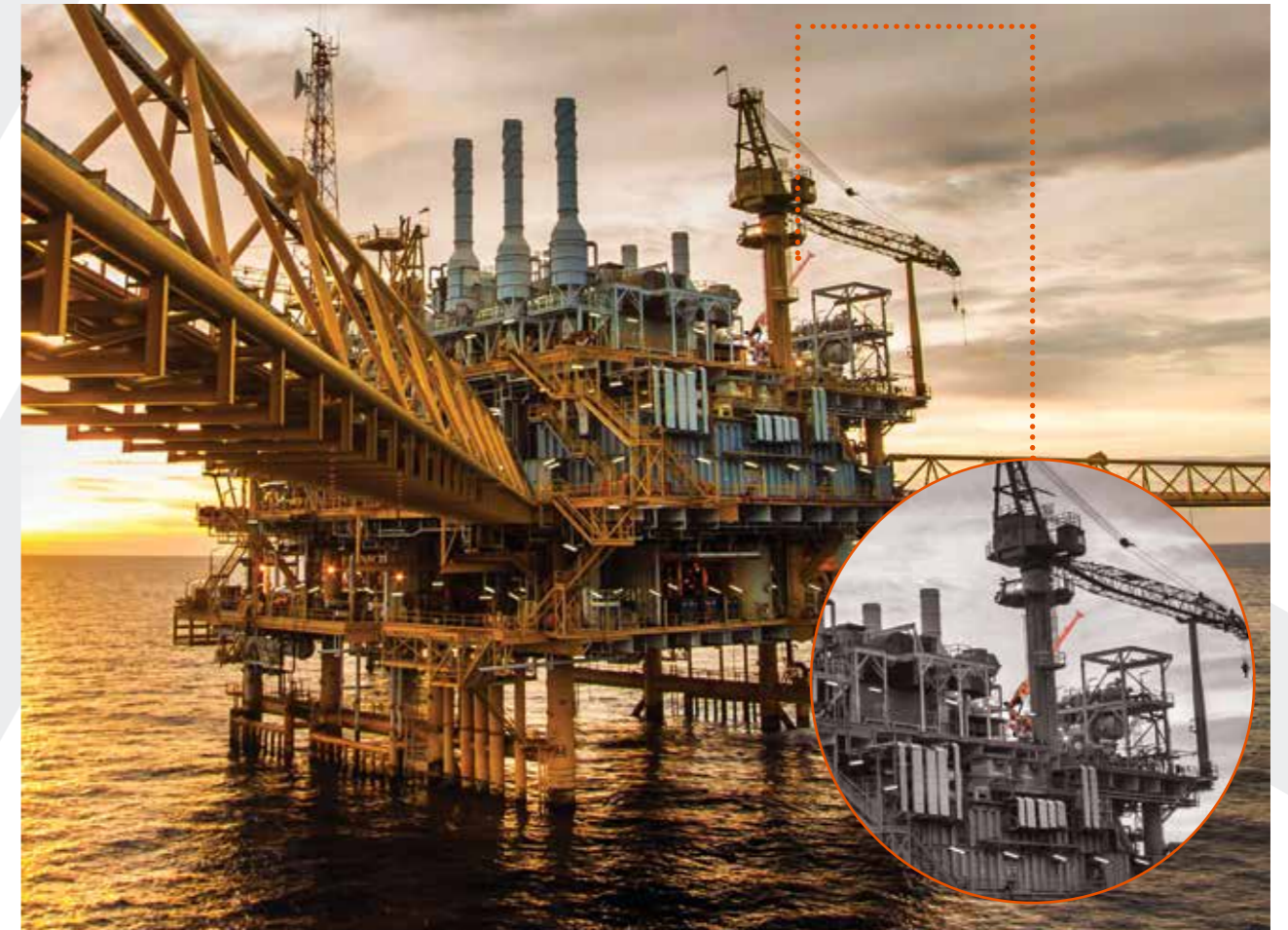
SPX312, working on an oil plant
