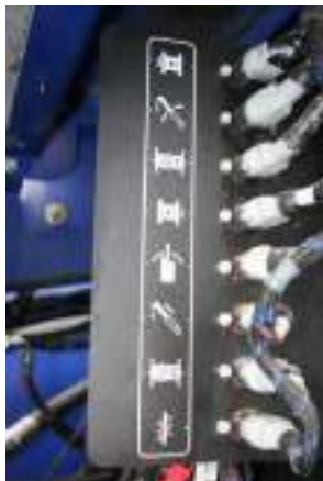
Emergency Back Up Bulkhead
