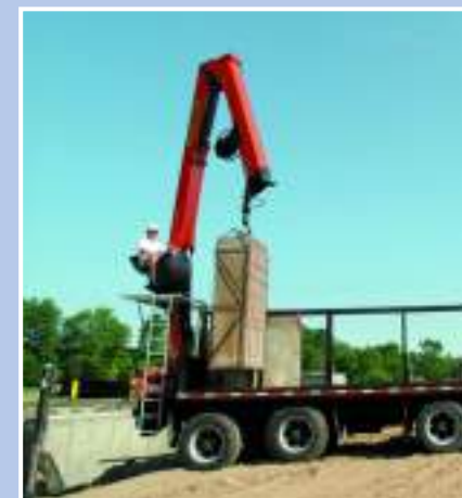
A high inner hook height allows the crane to reach and lift the 1st cage with ease
