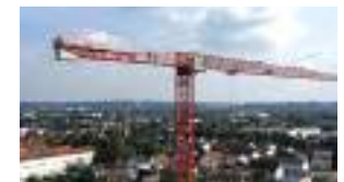
Raimondi MRT294 erected in Germany by Kwitek Krane
