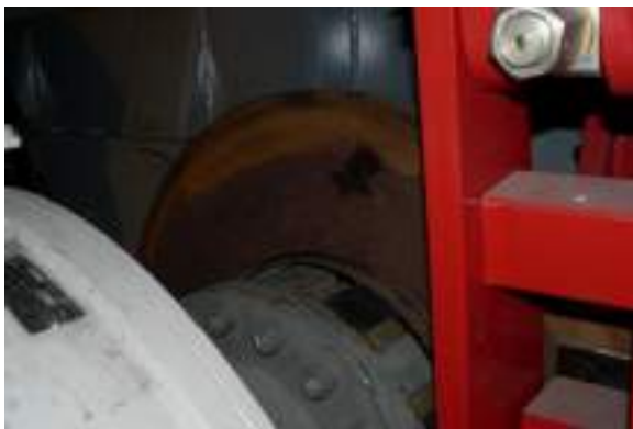
Figure 2-2: Oil dirt and rust on the brake disc must be removed
