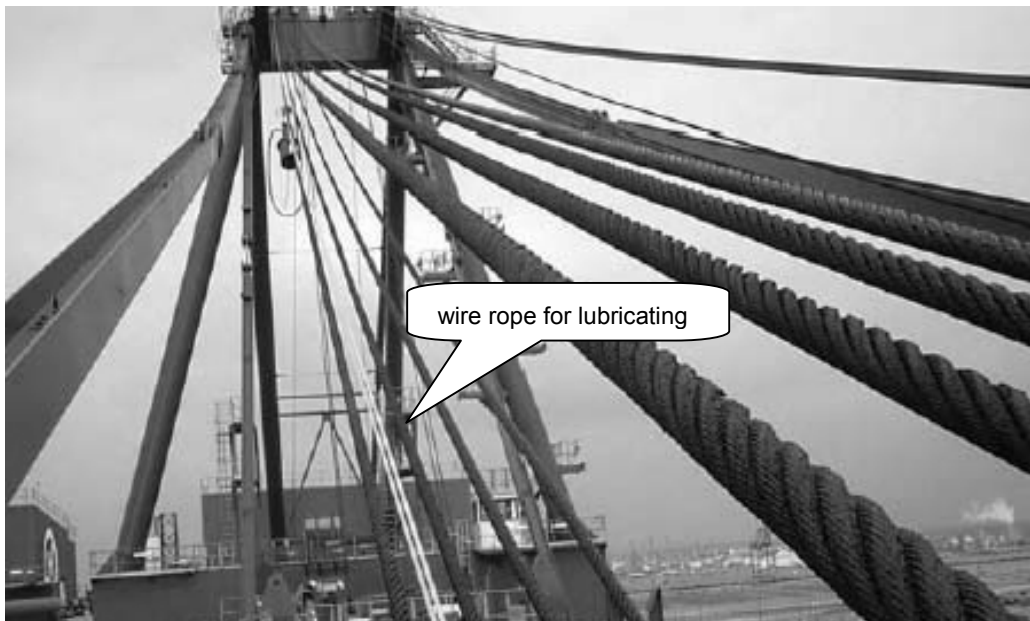
Figure 4-22: The lubricating of “dead rope” of boom hoist
