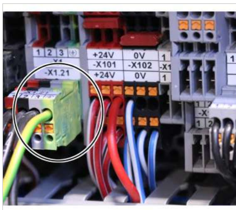
Bush multipoint connector in prong terminal block
