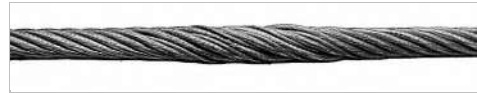
The joining of the wire rope has opened. The inner strands of the wire rope are visible.
