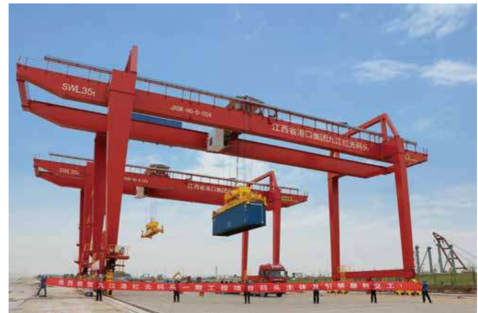
九江红光码头自动化轨道式集装箱门式起重机 Automatic Rail Mounted Container Gantry Crane for Hongguang Wharf in Jiujiang
